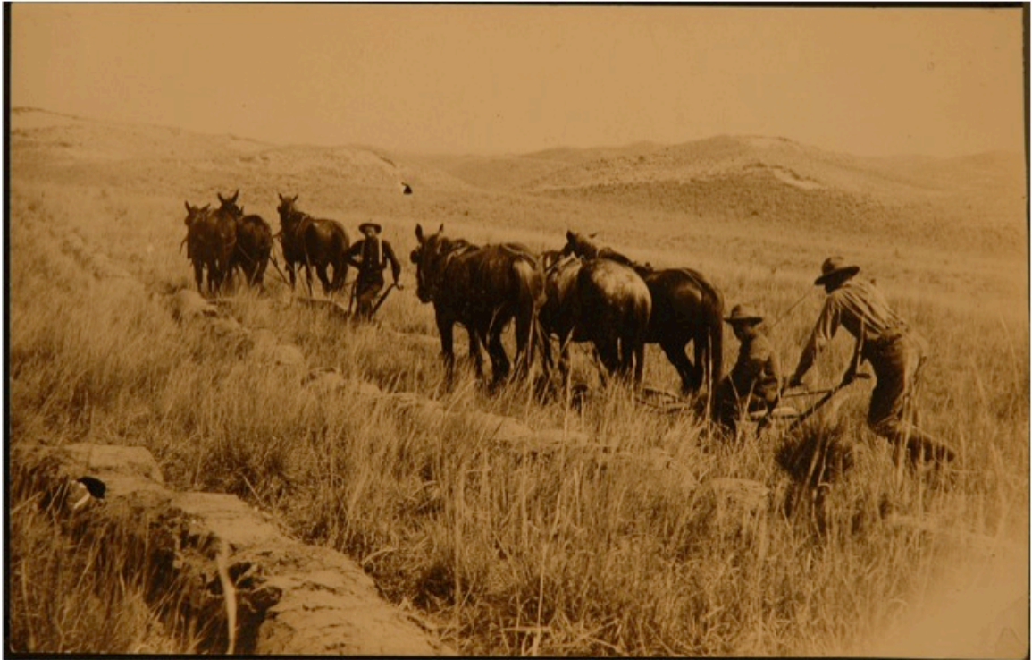
Figure 7 - Horse plowing and trencher operation. Source: USFS
